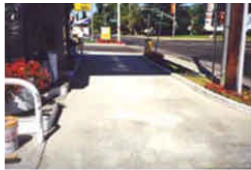
Lane After OIL-AWAY
